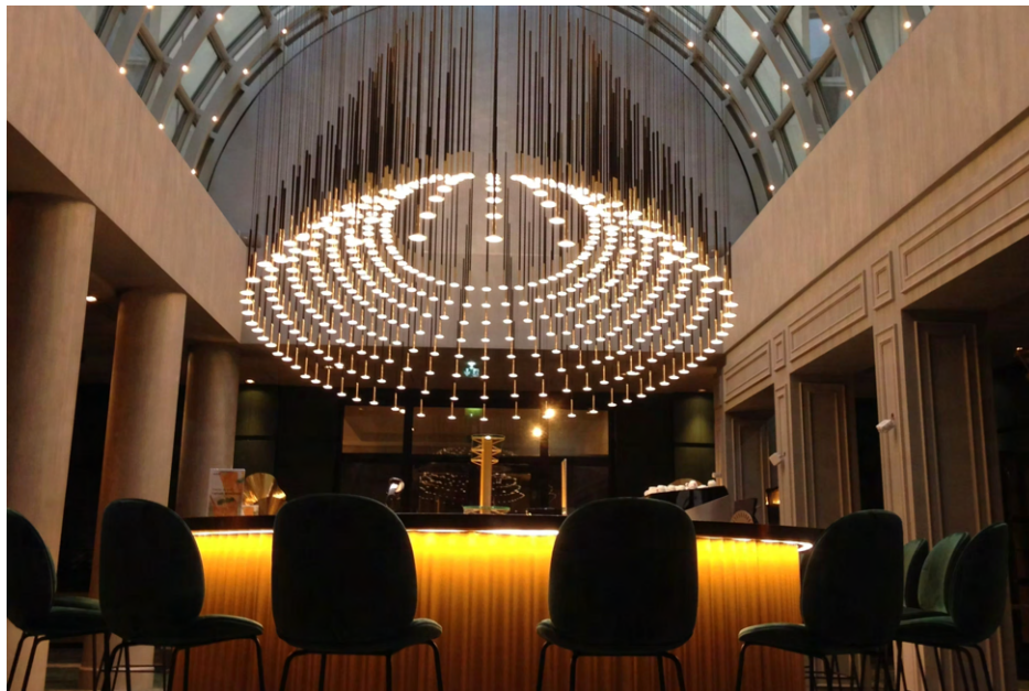
Figure 8.1: OLED lighting fixture. An OLED lighting fixture at Hotel Le Louis Versailles. Photo courtesy of BLACKBODY®.
