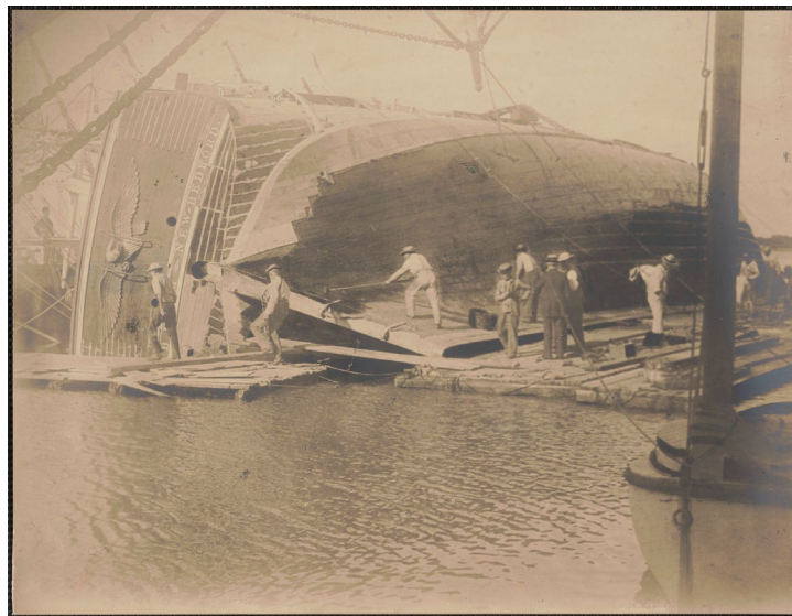
Figure 1.2.1 Aft end of the Whaling Vessel, Sunbeam, while hove down by Joseph Tirrell, 1850.
