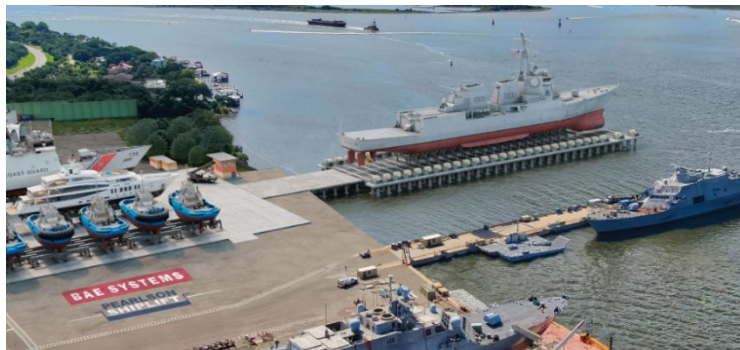
Figure 1.2.6 Rendering of a U.S. Navy destroyer sitting atop Pearlson’s 25,000 long ton capacity shiplift in Jacksonville, Florida.
