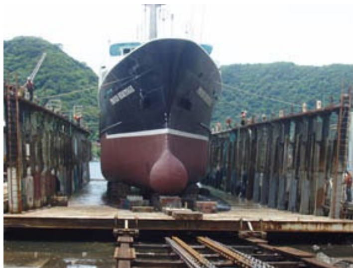
Figure 2.4.2 Crandall Marine Railway Dry Dock at Poga Poga, American Samoa. Notice the large cradle and the keel and bilge blocks that the vessel sits on. Additionally, the rollers, rails, and hauling chains can be seen in the foreground.
