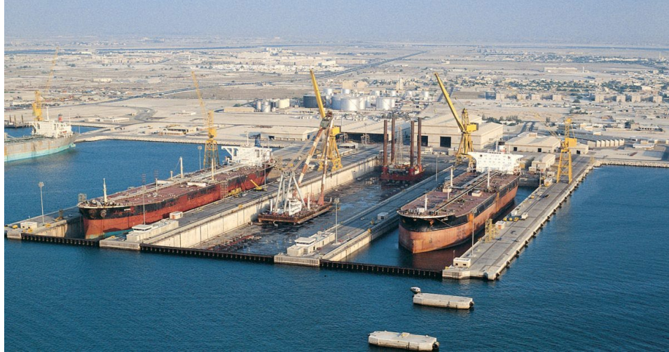
Figure 2.1.1 Three Graving Dry Docks in Various Stages of Flooding. Nauta Ship Repair Yard, Gdynia, Poland. ( https://www.gac.com/poland/shipping/dry-docking-support )
