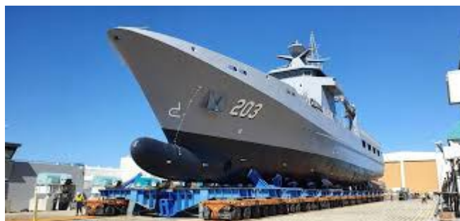
Figure 3.5.2: A Series of Hydraulic Lift Cars beneath Transverse Strongbacks supporting a
