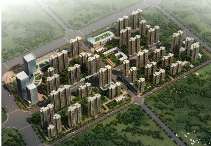
Figure 3-7. Aerial view of Shenglong. Source: Administration Committee of Zhengzhou Hi-tech Industrial Development Zone.
