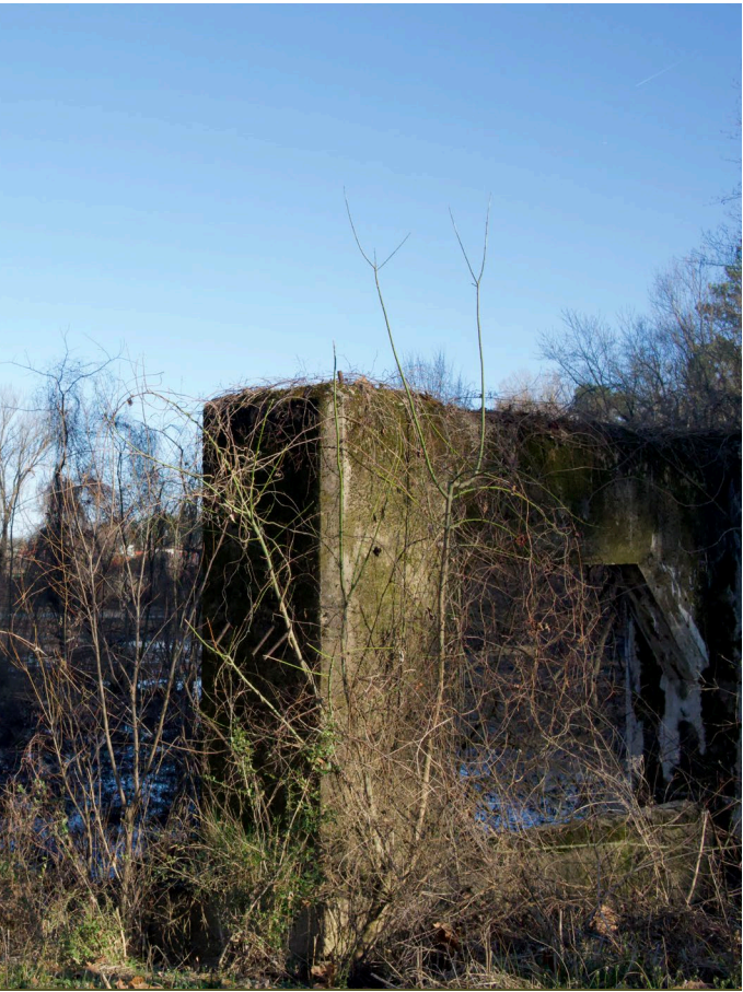
Macon Road bridge abutments at approximate location of Ell Persons lynching.
