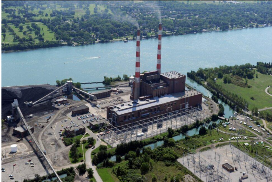
Figure 3: The TCPP when it was in operation (Fischer, 2024).
